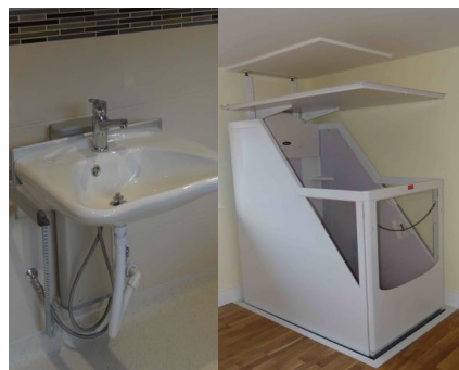
➤ Downstairs Assisted Bathroom: Height adjustable Wash Basin. Through Floor Lift from ground to first floor
