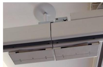
Our unique gate system fitted to ensure the tracking is correctly lined up when transferring between multiple rooms and pieces of ceiling track
