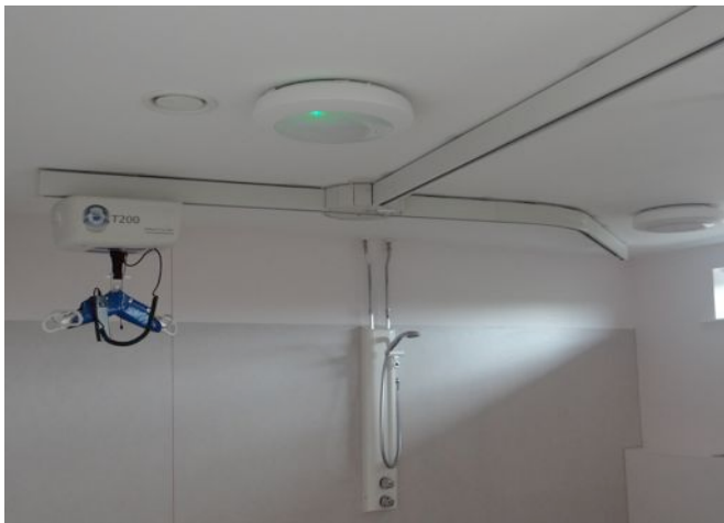
The turntable allows the hoist to run in several directions, and the 18 possible exit points achieve exact positioning over the WC or changing bench. The turntable is operated automatically by the hoist, so the carer never has to leave the patient's side to operate a switch
