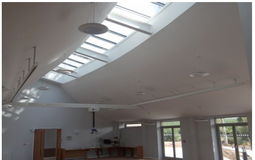
OT200 Ceiling Hoist on large H system in Lounge. The H System measured 6m x 13m and was installed on a curved roof. Even on a system of this size the OT200 glides smoothly and with little user interaction
